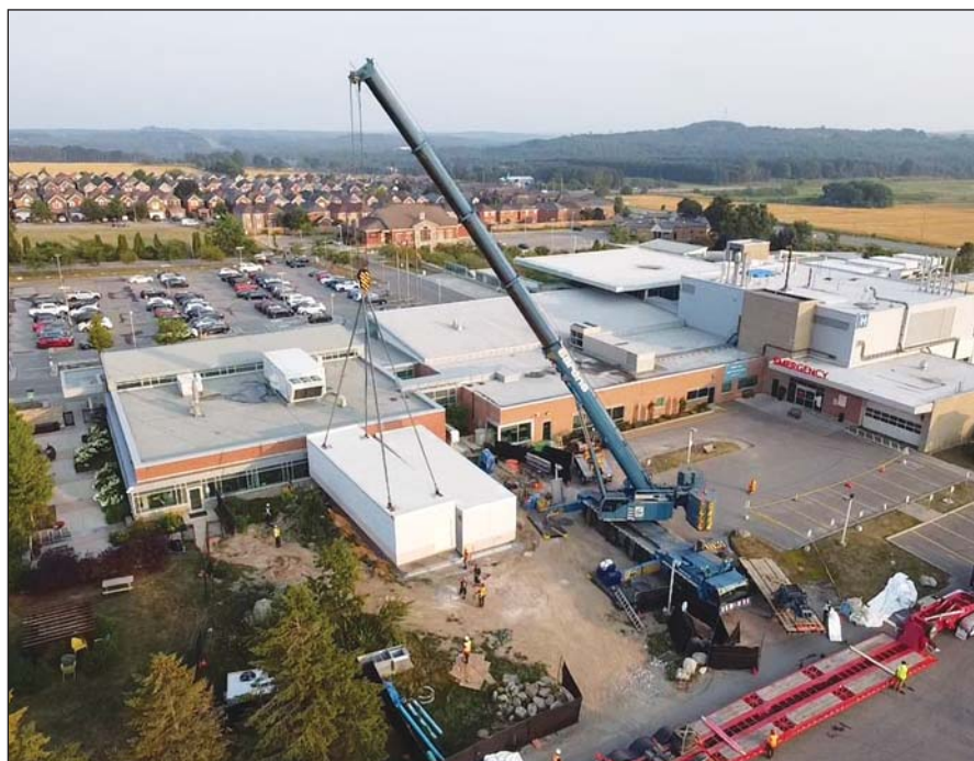
A cassette for diagnostic imaging is craned into position at Headwaters Health Care Centre, August 2025.
